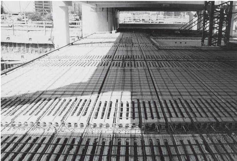
*Fig. 4.16 Slab end prepared for casting of a fairly large corrugant flange*
