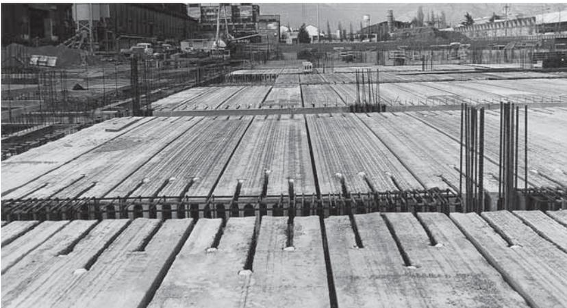
Fig. 4.9 Floor in continuity on several supports:
