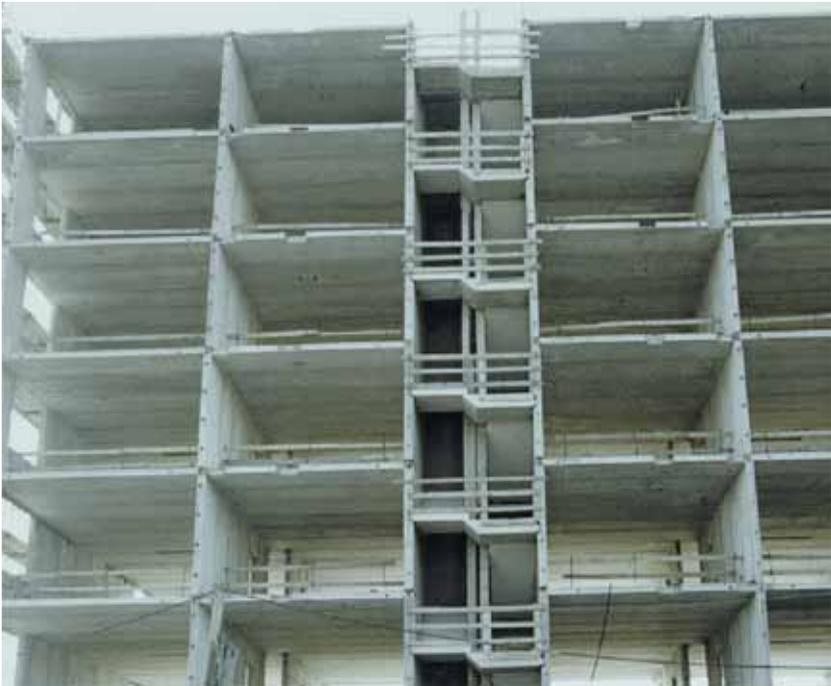
*Fig.1.4 Hollow core bearing walls and floors in a multistorey residential building*
