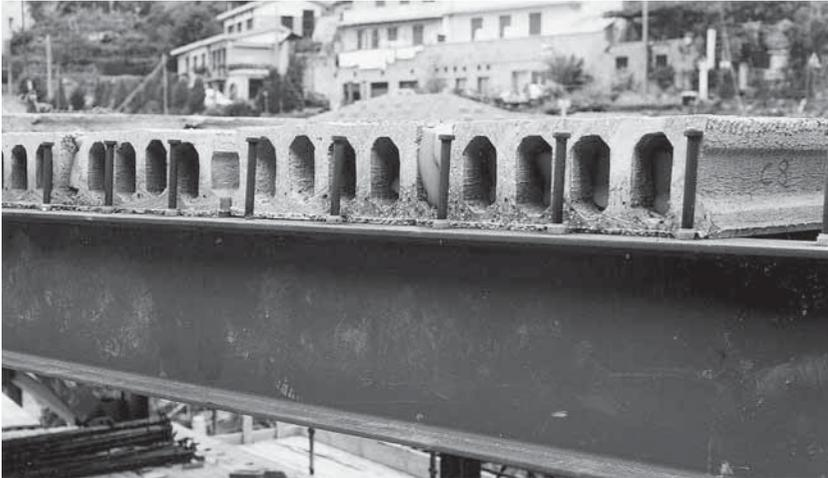
*Fig. 4.22 Hollow core floors on steel beams.
