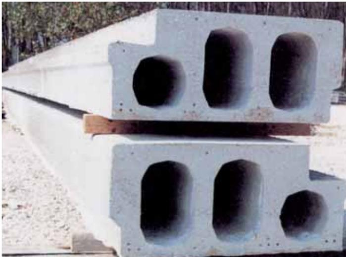
*Fig. 2.7 Slip-formed slabs with widened webs or special shaped webs (grandstands for a stadium)*
