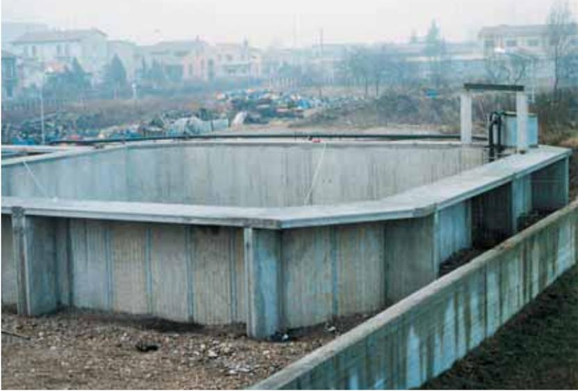
*Fig.1.3 The hollow core walls of a water treatment tank*
