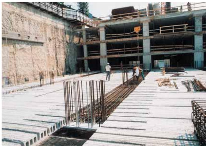
*Fig.1.2 Hollow core slab floors in a multistorey underground parking garage*
